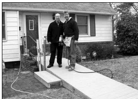
East Meadow President Dr. Alan Alterman (l) and IPP Jay Steinmetz (r) stand on nearly completed ramp during a pause in construction.
